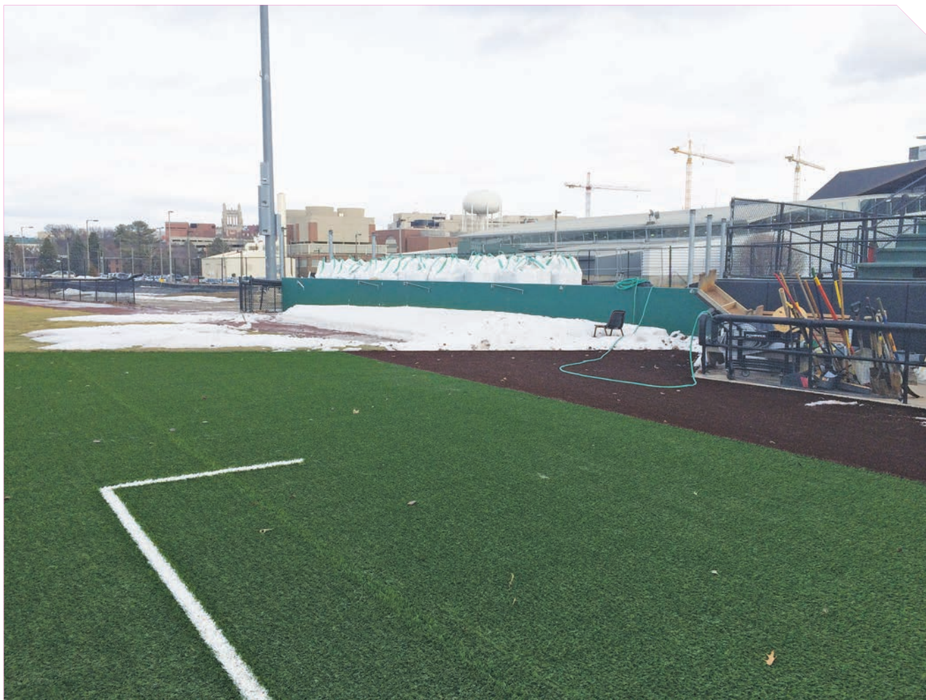
Spring 2014 after Phase 1 should have been completed. Because winter hit early in 2013, the turf was installed but all of the infill still had to be placed before spring ball.
