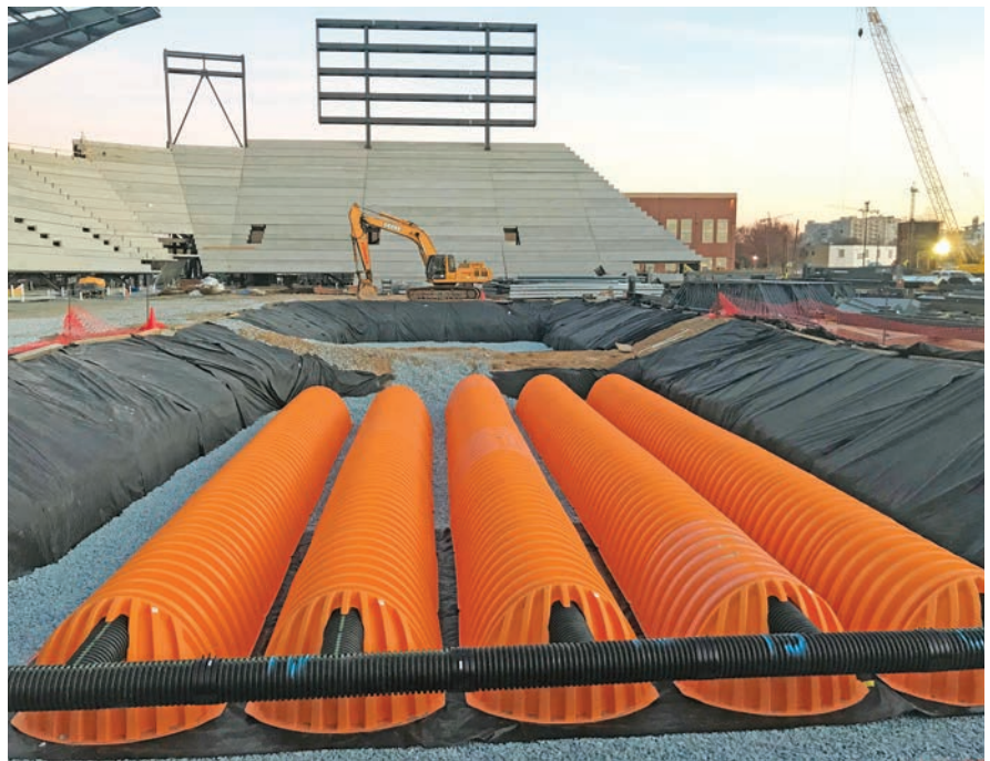
The storm water storage system used these chambers from ADS to handle the capacity spec of 50,000 gallons.
