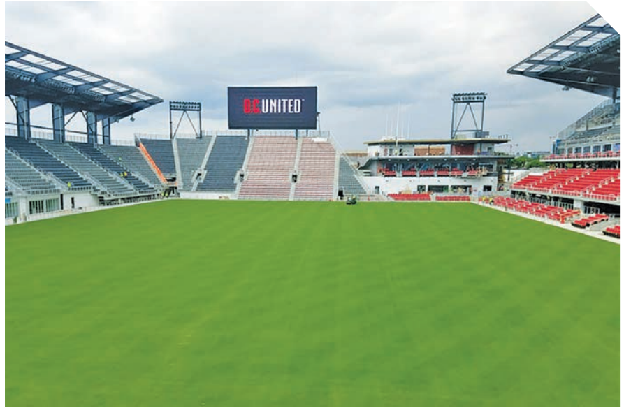
The completed field with five storm water storage units and a network of pipes for drainage and sub-irrigation.
