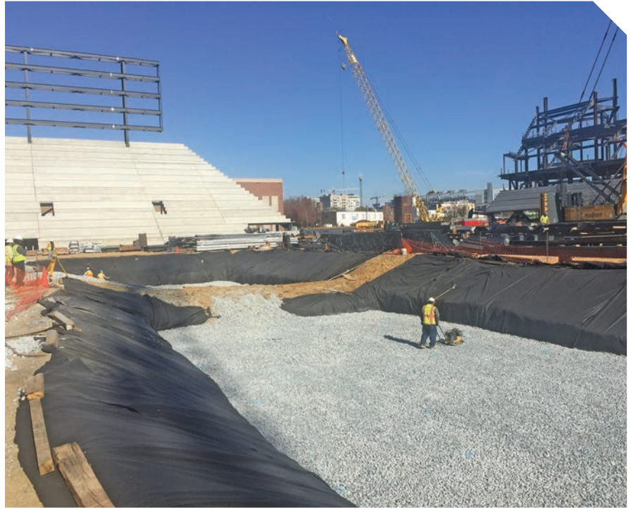
A stone bed was put under and around the eight chambers, which were also wrapped in geotextile.
