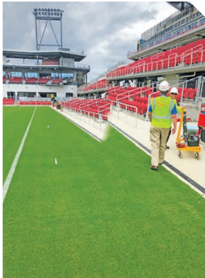
The Magnolia Construction team does its last onsite inspection before the first game.
