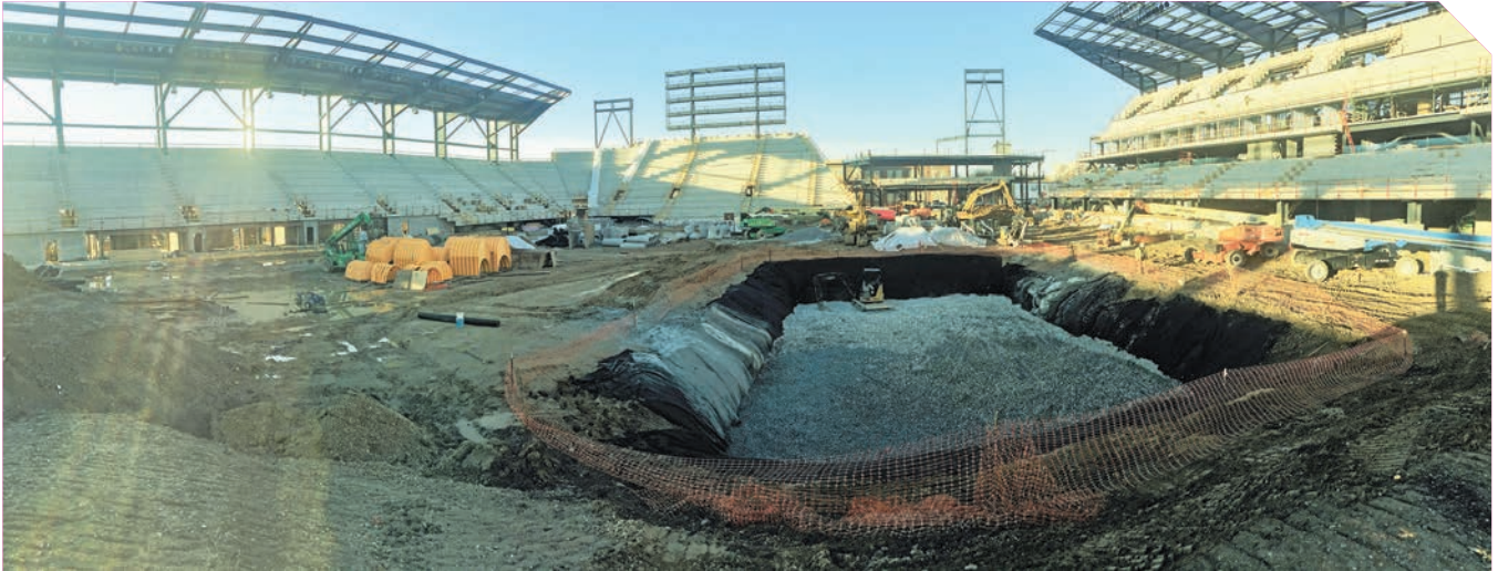
Space was tight during construction of the new $500 million D.C. United Audi Stadium.
