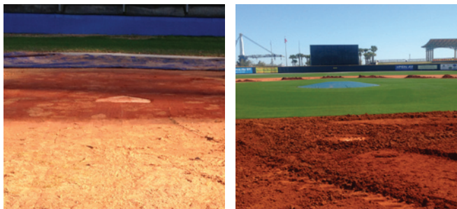
▲ Left: Leveling home plate with mound clay at Stone County High School, Wiggins, MS. Field maintained by head coach Hayden Cox. Right: Adding clay to the Pensacola Blue Wahoos Field, Pensacola, FL, where Ray Sayre is head groundskeeper.
