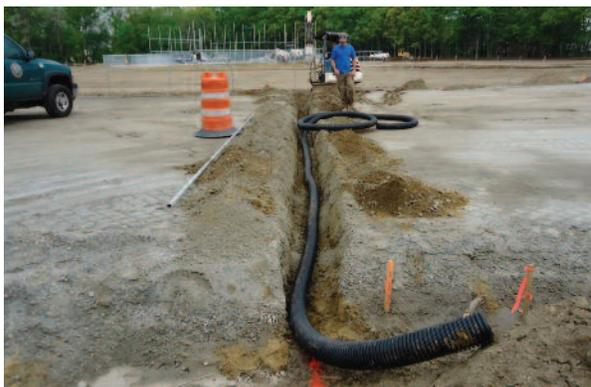
bottom of the trench typically are lined with a suitable drainage filter fabric. Normally a French drain does not include a pipe; however, the inclusion of a pipe makes this type of drainage system more efficient.
