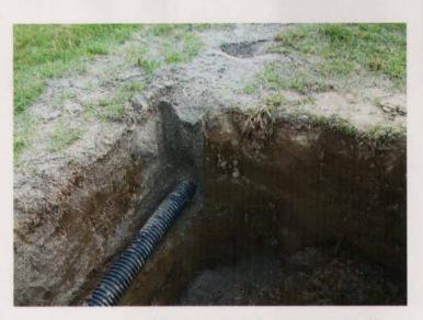
migrating into the pipe. The Greenshield Systems uses a 2-inch corrugated perforated pipe with small slits eliminating the need for a sock. A geotextile sock around a pipe works great if it does not have soil contact or become clogged with fine particles. A sock can be used to protect a pipe with larger perforations from sand migration and the sand backfill protects the sock by stopping the fine particles.
