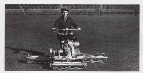
ere we have an example of one of the first gasoline powered triplex mowers used on sports field maintenance. This is a Toro Triplex mower used at the Rose Bowl in the 1920's. Innovations such as the powered triplexes, which we take for granted today, were not always around. The horse drawn mower was the only method available until companies like Toro, National and Ransomes incorporated internal combustion engines to the machines.
