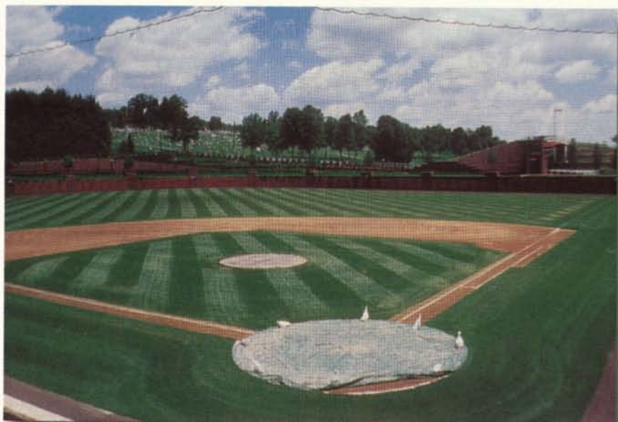
The field is located on what used to be a farm field. The native top soil was removed during construction, then backfilled with topsoil augmented with compost.
