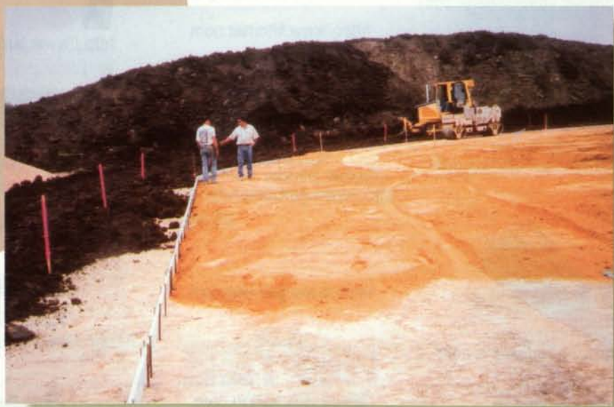
The skinned surface of the infield was 60-70% clay and 30-40% sand, with calcined clay incorporated to a depth of one inch.
