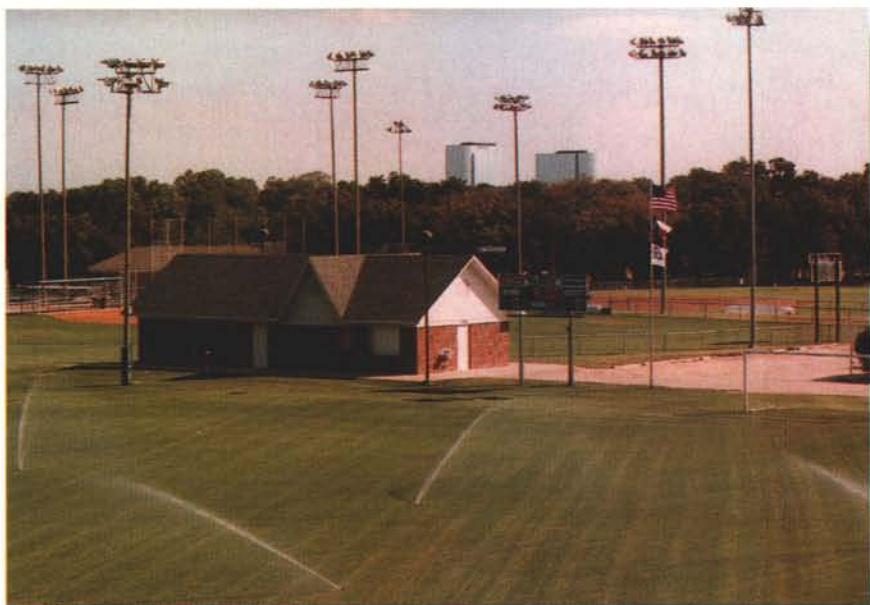
State of the art lighting and irrigation systems were installed at the complex in 1988. Field 5 is lit by four 45-foot-tall poles supporting five metal halide lamps each. Courtesy: City of Farmers Branch
