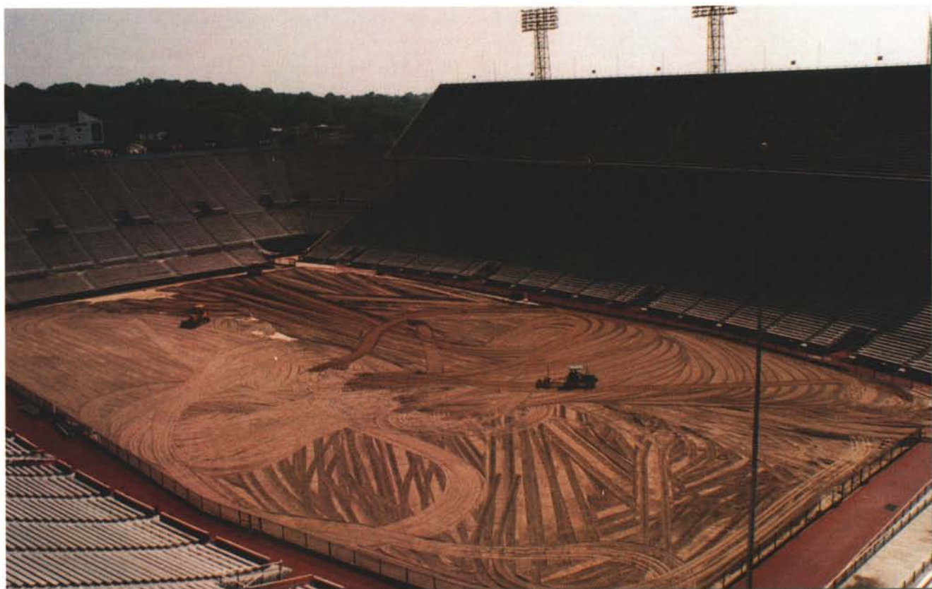
Renovations in 1999 created a 90 percent sand base that increased infiltration and percolation rates and eliminated the 4-inch organic layer.
