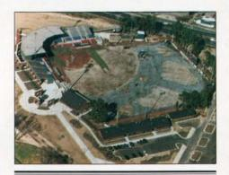
Because it has no underground drainage, the Golden Park field was laser-graded four times, and a high percentage of sand was added to the soil profile.
