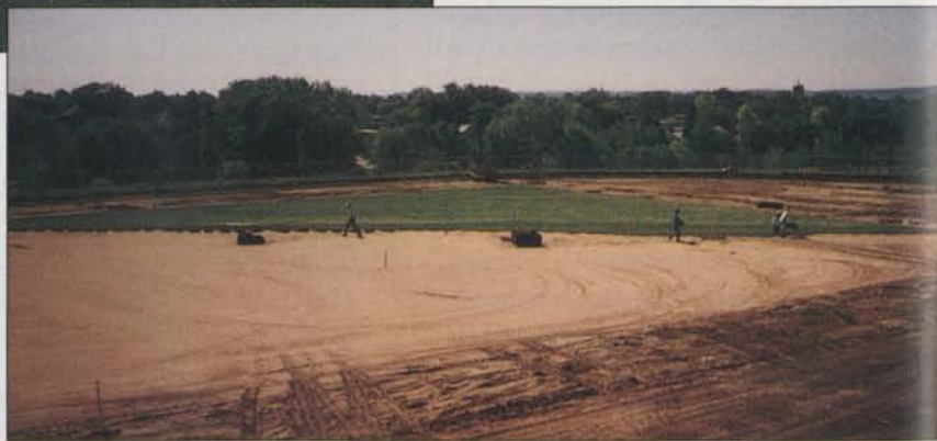
Wayne Klosterman (right). Prefabricated drain tubing was connected to eight-inch collector lines on the side of the University of Dubuque football field. Bluegrass sod on a peat base was installed in late June.
