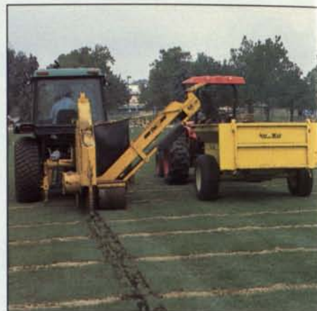
Installation of the sand-conduit drainage system, July 1994.
