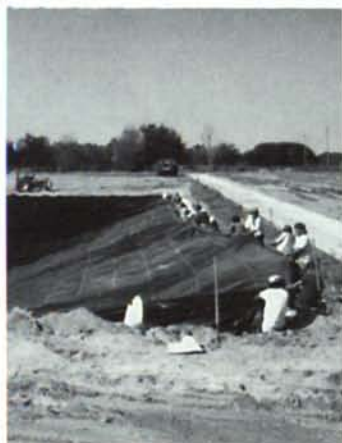
STORMWATER RETENTION POND
