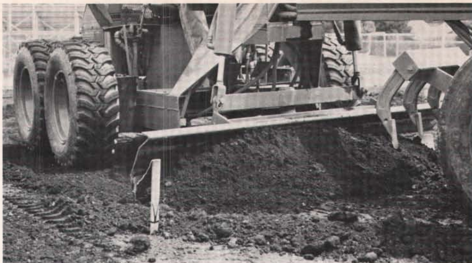
Stakes indicate both the subgrade and the finished elevation.
