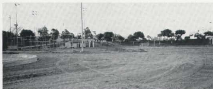
Park roughly graded prior to installation of drainage, subirrigation and sand.
