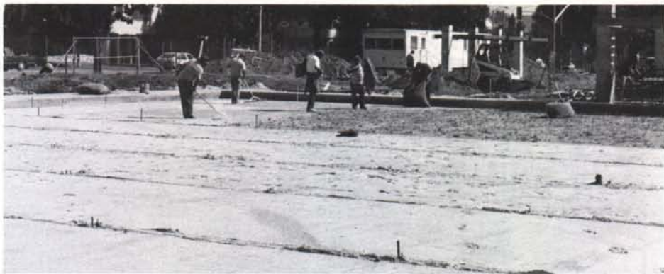
Sprigs of Tifgreen hybrid bermudagrass are scattered across the sand greens at Roxbury Park.
