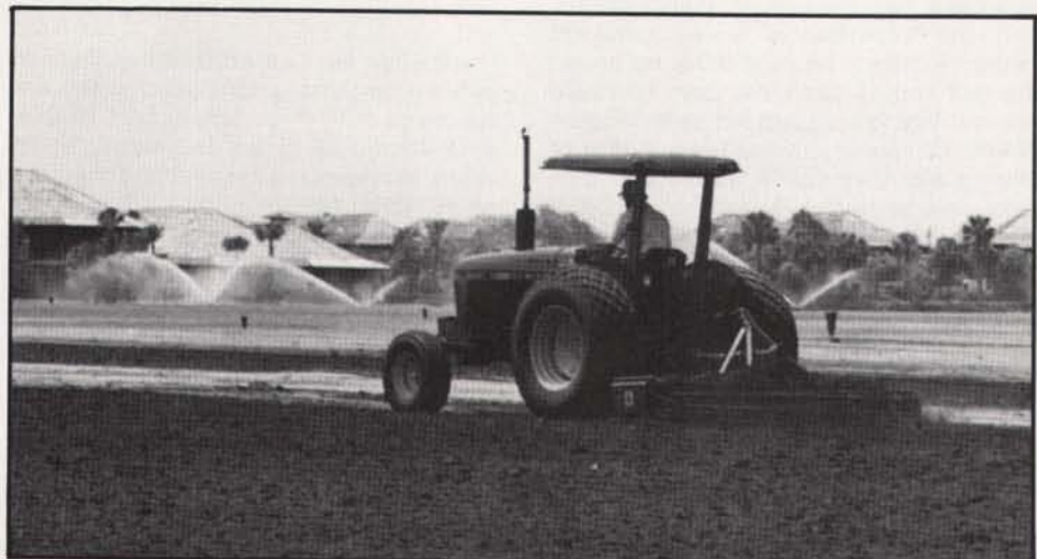
All fields are topdressed with sand and smoothed with a box scraper prior to fertilizing and irrigating.
