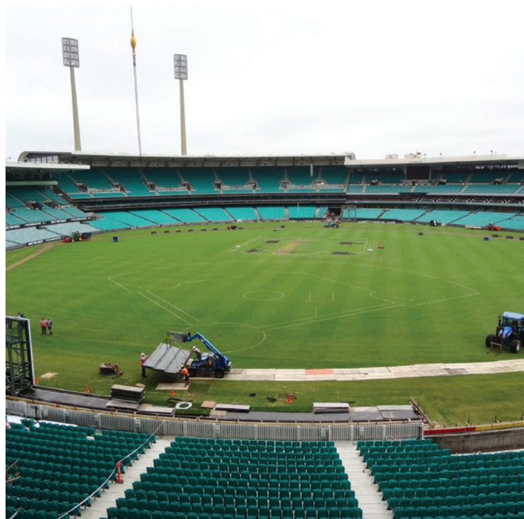
▲ Laying out field and first harvest of sod from warning track area.
