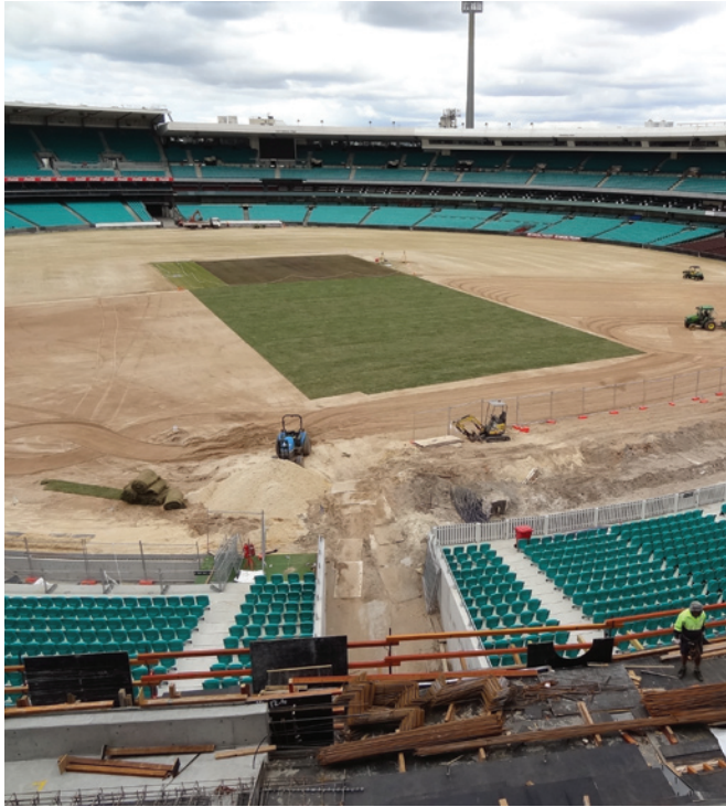
◀ October 2013 renovation of leveling area where infield would be placed.
