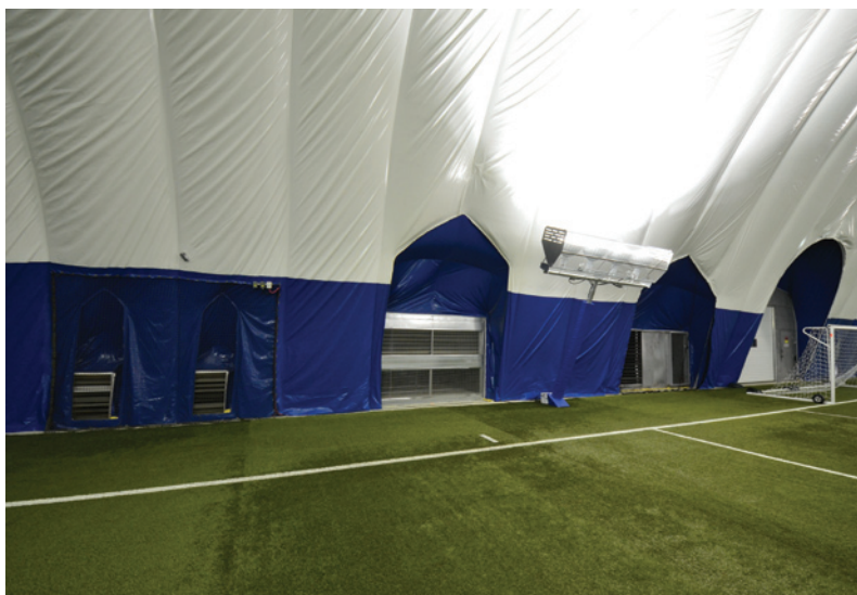
▲ Interior view of fabric connections for mechanical equipment and vehicle airlock (King City, ON).
