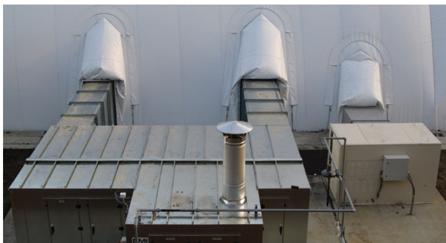
▲ Main heat and inflation unit and standby inflation fan (Greenville, PA).
