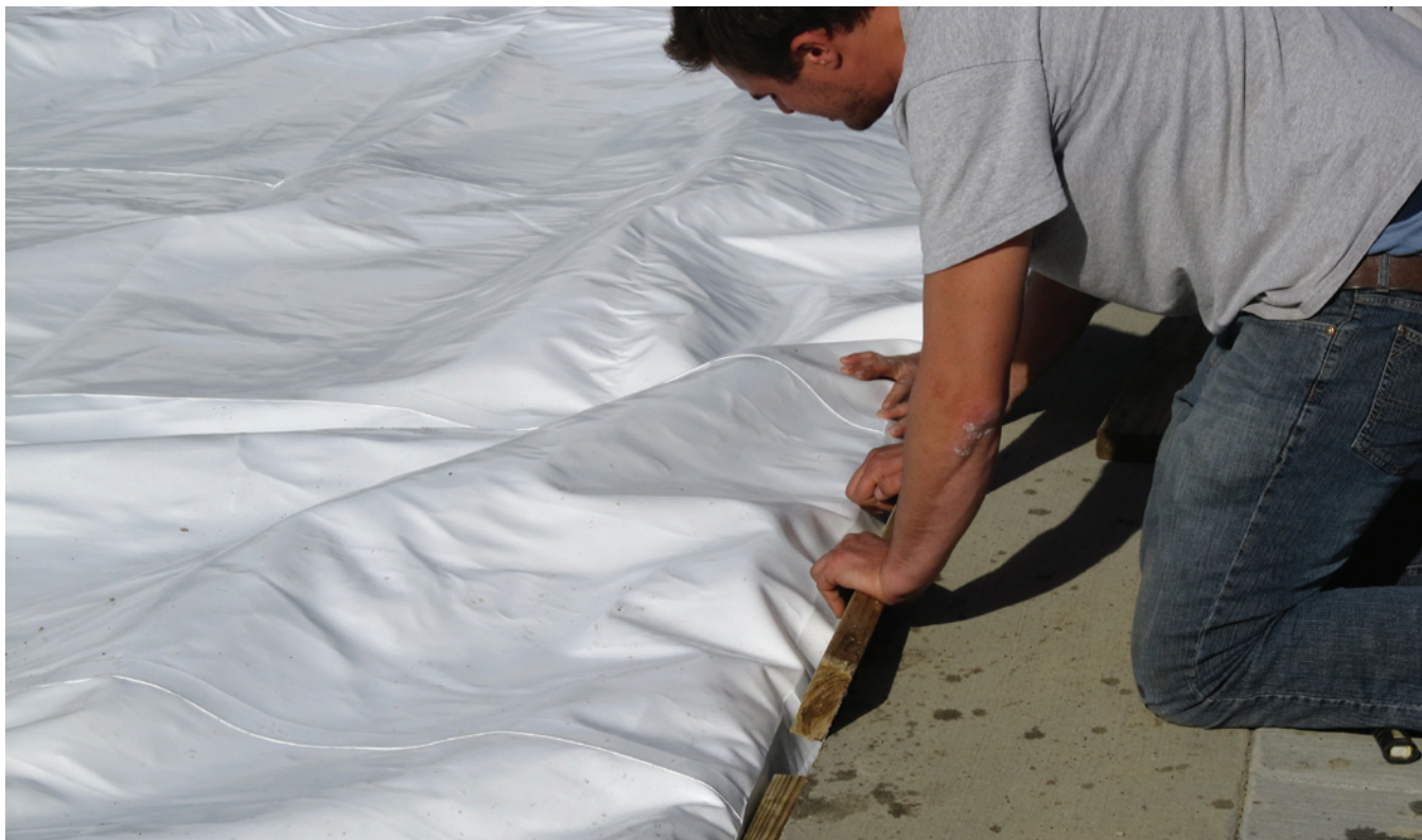
▲ Fabric membrane being locked into anchoring system (Greenville, PA).
