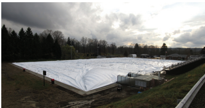
▲ Dome spread out and connected to the grade beam, beginning inflation (Greenville, PA).
