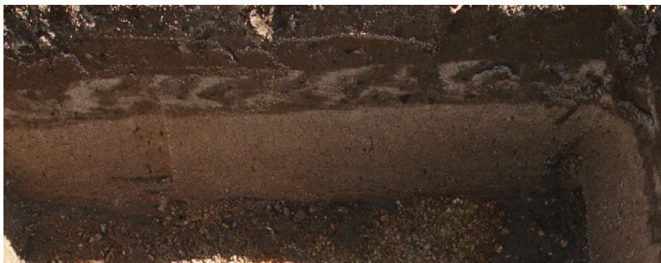
▲ Layering in a sand-based system caused by a buildup of organic matter. Image courtesy of Nick Fedewa.
