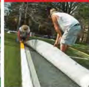
Loose-laid narrow seams over stone
