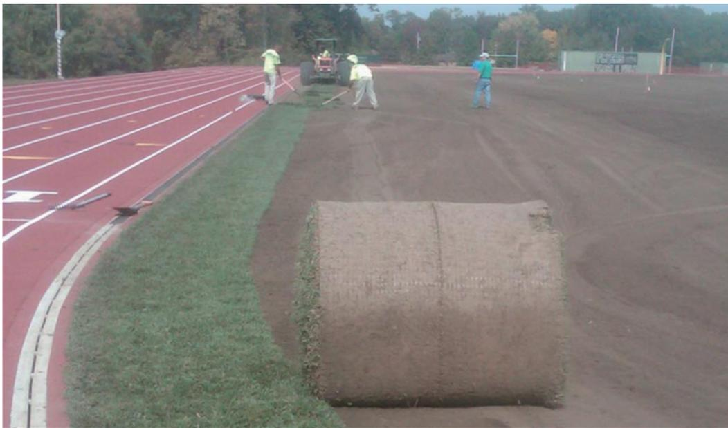
We brought in a lot of soil and ran soil tests and we were focused on organic matter content and were hoping for at least 2.5-3% which we were able to find, the pH was where we wanted it but the core chemistry needed some help.
