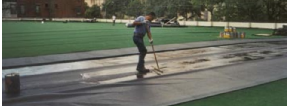
>> ADHESIVE being applied for a total gluedown with a stand-up squeegee.
