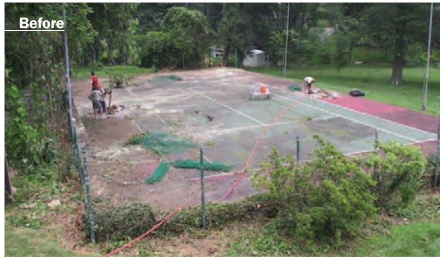
>> TURF IS BEING USED to cover cracked courts and make them playable again without total reconstruction. These before and after illustrate such a transformation. Photos courtesy of Pro-Sport Construction, Inc., Devon, PA.
