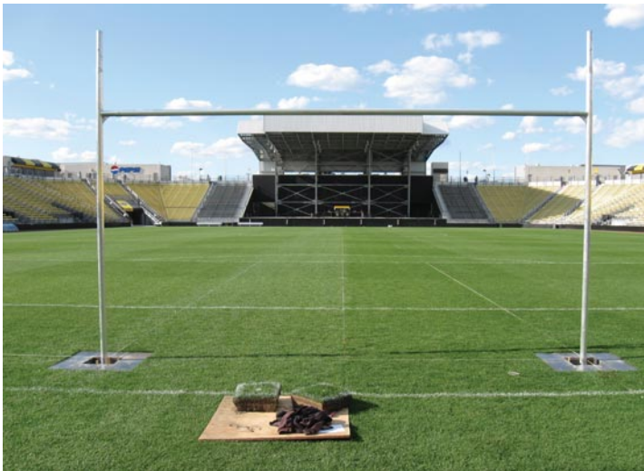
Above Left: Only the two squares of sod were removed for rugby; here is first set of posts in south end. Above right: Halfway done with rugby stencil. Due to the high temperatures, we had to work through the night into early morning to prevent stencil burn.
