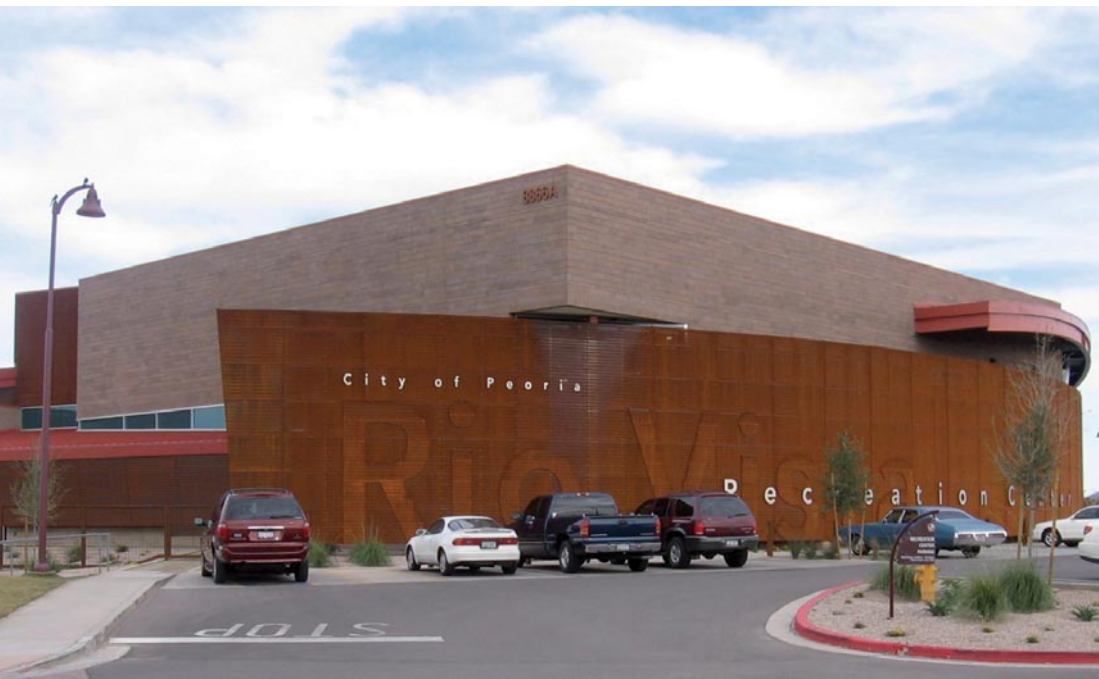
» THE MAIN BUILDING and gymnasium at Rio Vista Community Park, Peoria, AZ.
