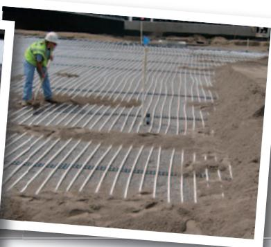
Target Field would then become one of the only MLB stadiums to have a state of the art **hydronic heating system** which was designed to accommodate the seasonal shading of the field.
