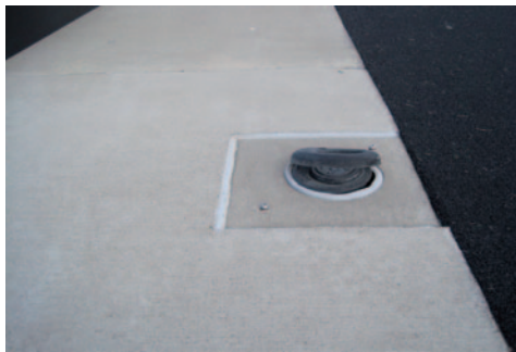
» LEFT: The old heads had heaved because of frost. MIDDLE: I-25 warning head running as Underhill M-160 head comes on. RIGHT: Large heads come on.
