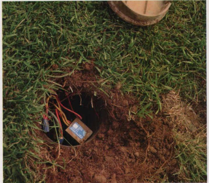
Underhill decoders are attached to every valve and irrigation programming is relayed to each valve over the two-wire system.
