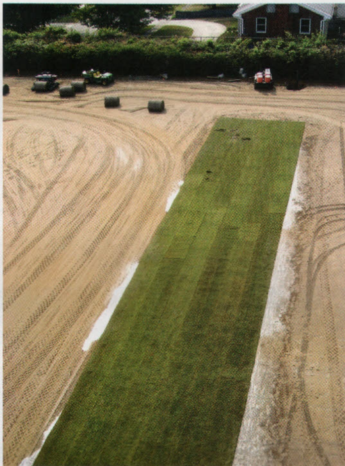
Here's a shot from construction of the University of Kentucky's football practice field. Courtesy Jeffrey L. Bruce.
