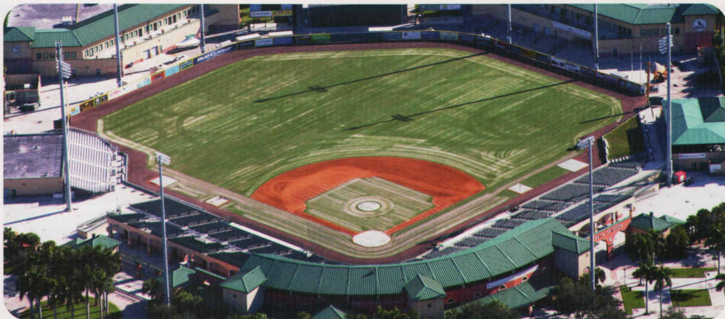
From the complete renovation at Roger Dean Stadium in Jupiter FL, spring home of the Marlins and the Cardinals. This shot shows the new Celebration bermuda turf just after installation during the first topdressing. If you look closely you can see the guy in motion putting out the 90/10 USGA mix. Picture taken by Sports Turf One VP Bill Gillan; pilot was Dell Haverland.
