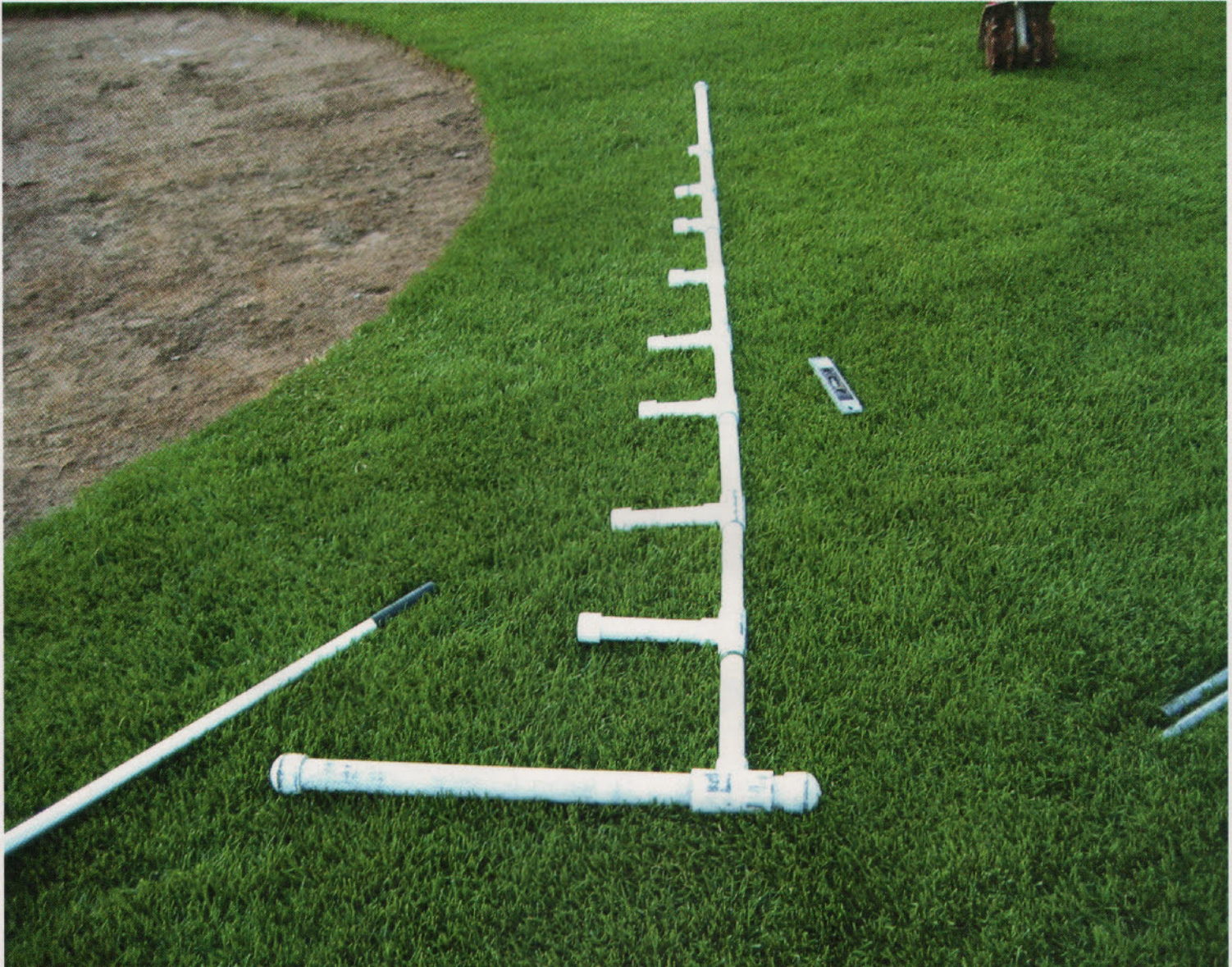
The author's homemade tool that helps in getting a 1-inch drop per foot when completing the front of a new mound.
