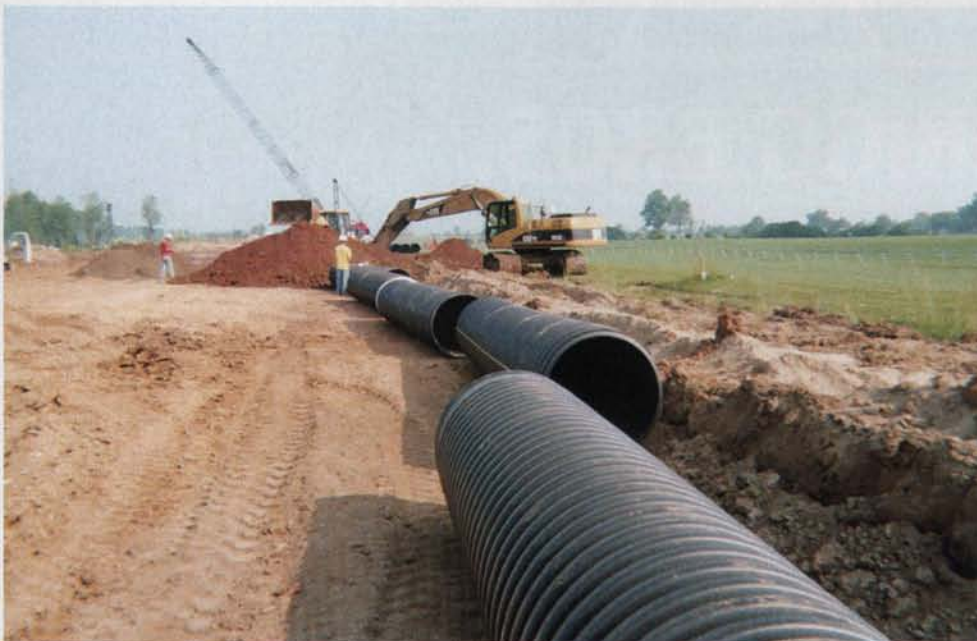
Elevating the grandstand apron required an end-to-end drainage structure to empty the runoff of the trench and roof drains.
