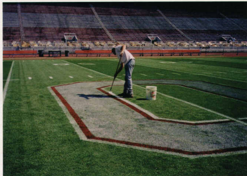
The crew at Ohio Stadium paints the second coat of the white border around Block O with a 4-inch roller using Pro-Stripe Super White.
