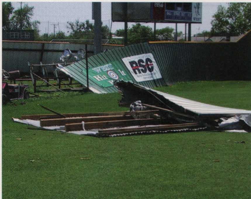
A May tornado destroyed two storage buildings and blew them onto the field, where they were pulled off with a tractor.
