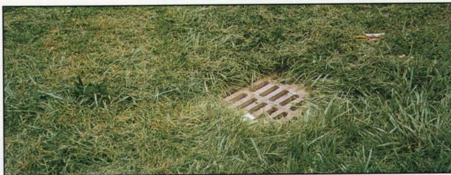
A hidden sewer cap on an athletic field can lead to a series injury and potential lawsuits.
