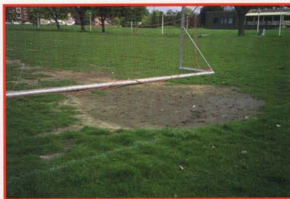
Depressed surface grading, destroyed soil structure and compaction: a classic example of integrated drainage problems. Photo courtesy: LANCO Amenagement Inc.
