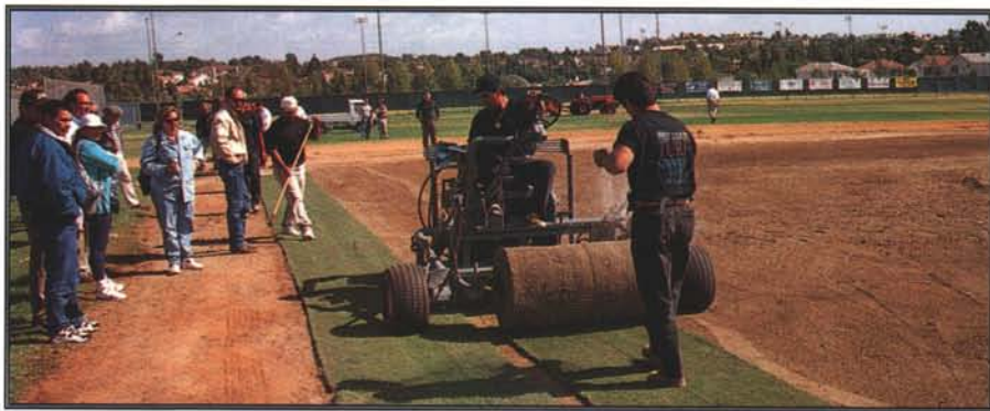
This machine helps lay big-roll sod. Courtesy: Trusty & Assoc.
