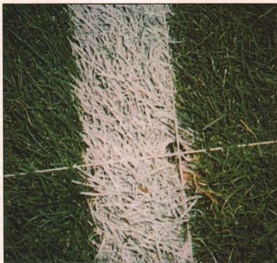
Crossing two string lines allows paint crews to accurately line the field and center the logos.
