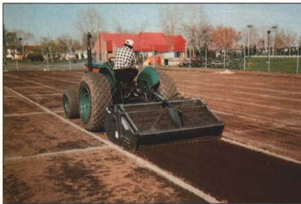
Installing modern slit drainage in new field constructions is a very straight-forward and quick process. Courtesy: Lanco.
