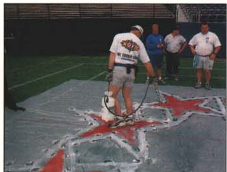
The crew used hand-held compression sprayers for fine detail work on the field's logos. Courtesy: Steve Wightman.
