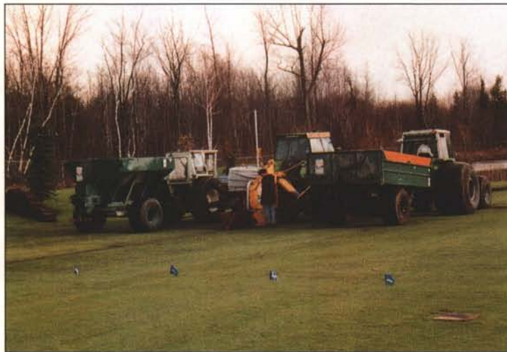
Modern slit drainage equipment limits installation time even in existing fields by simultaneously cutting, excavating, and filling slits in one pass. Courtesy: Lanco.
