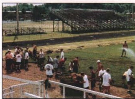
This football field reconstruction project was completed at about half the usual price because of community participation. Volunteers included members of the football team, who turned out to help lay the sod they would play on. Courtesy: Jim Puhalla
