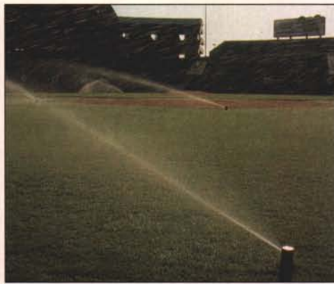
Install sprinkler heads that have very strong retractable springs, a small top size and a protective covering.
