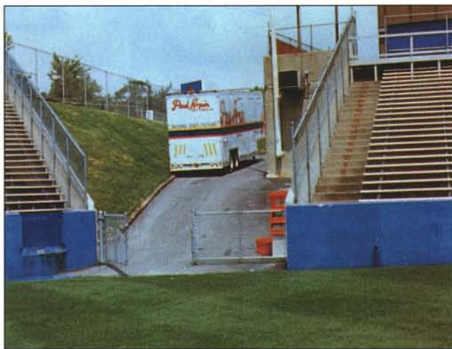
In older facilities like Foxboro Stadium, steep, narrow accesses have contributed to compaction and erosion problems. Photos courtesy: Steve Guise.
