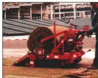
INSTALLED CLEVELAND INDIANS IN 42" AND 48" ROLLS
