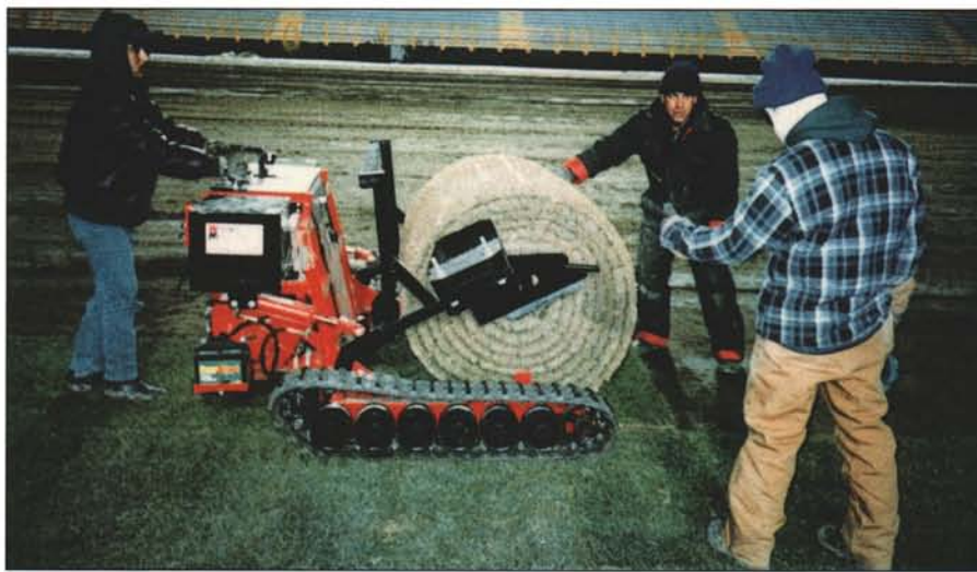
With the temperature below 10 degrees, the crew started laying sod minutes after the first heated trucks of sod arrived from Maryland. Photos courtesy: Jack Kidwell.
