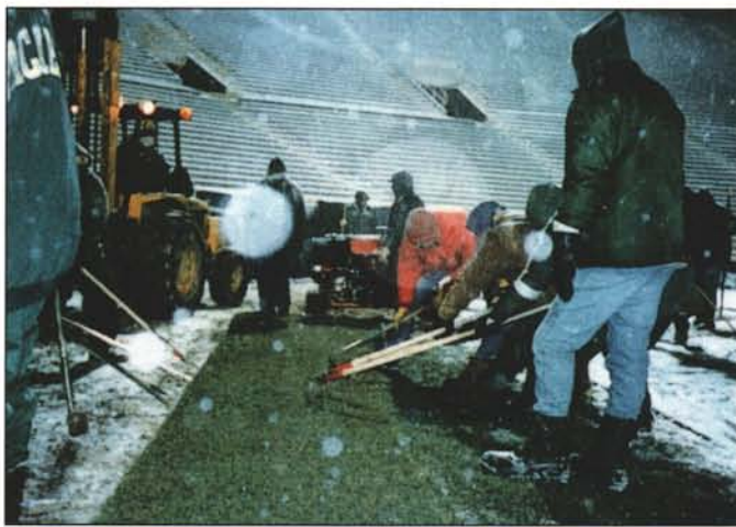
Finishing up the job in a driving snow storm, workers move a tarp in as the last strip of sod is pulled up and rolled.
