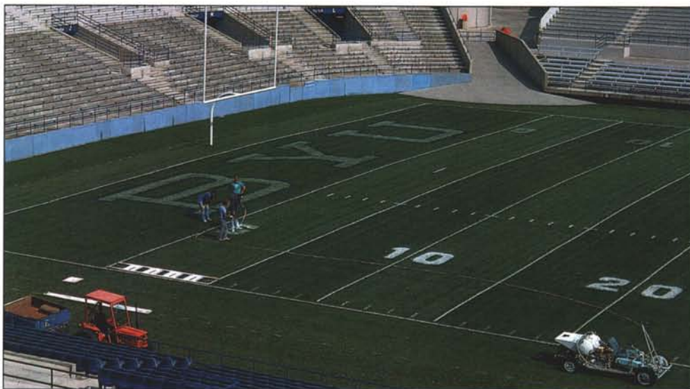
After painting numbers and hash marks, the paint crew will move into the end zones and paint the "BYU" letters.
