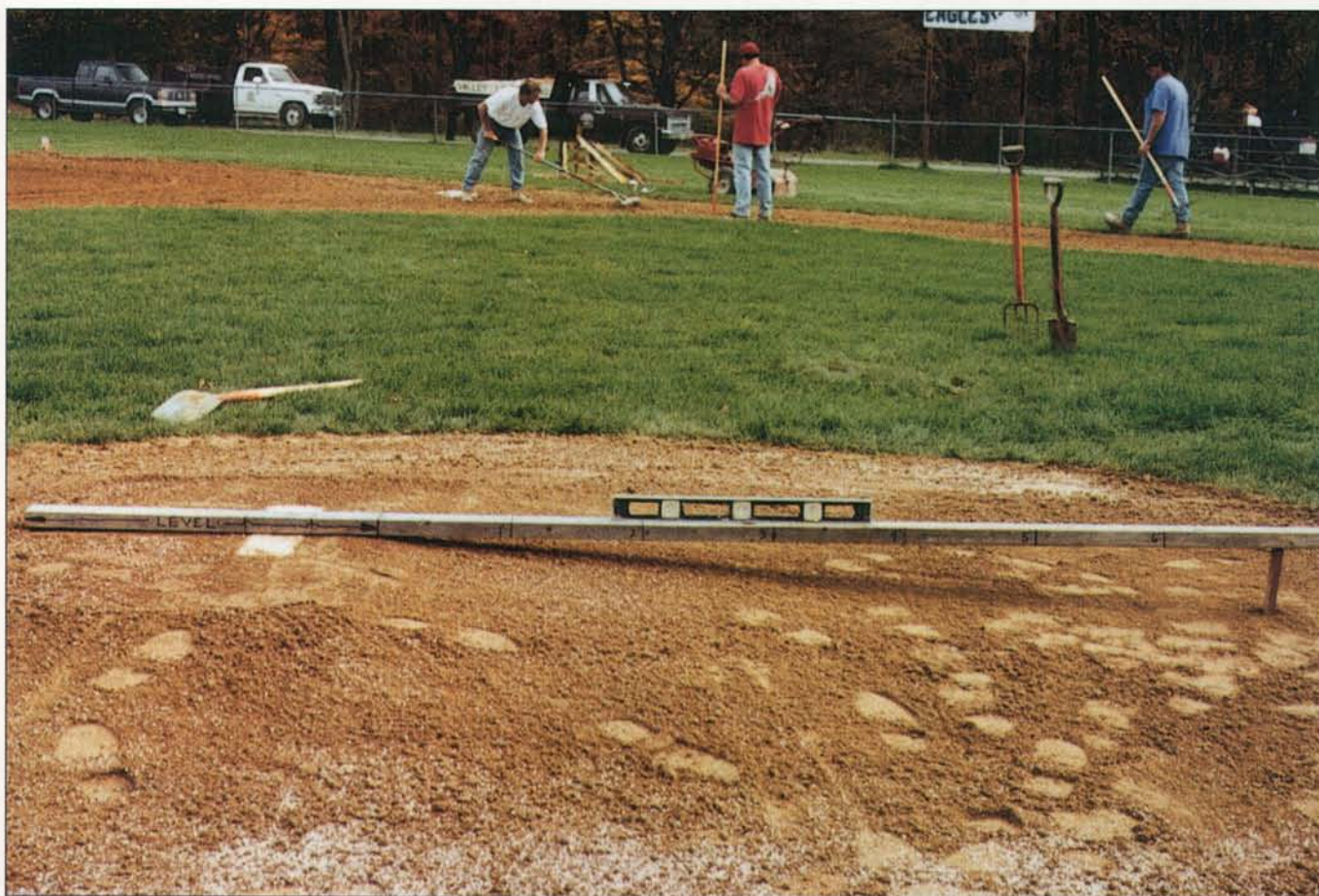
Using a ten-foot-long board, you can make a regulation pitcher's mound.
