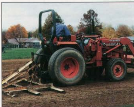
A level bar up to ten feet wide helps get a smooth, consistent surface. This one was easily made in the contractor's shop.
