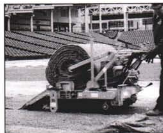
INSTALLED CLEVELAND INDIANS IN 42" AND 48" ROLLS
